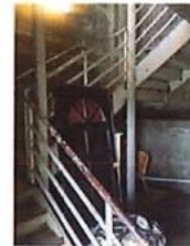
Fire Training Tower
